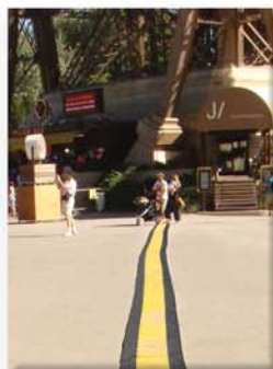
... in Paris, France, protecting cables running under the Eiffel Tower
